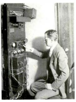
The amplifier operator in a recording studio has ready control of the overall loudness of the record
