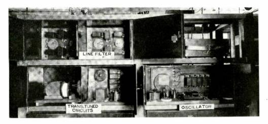
For the experimental installation of high frequency carrier telegraph at Maumee the apparatus was installed in steel boxes. This illustration shows the sending apparatus
