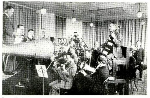
To record by the old acoustic method it was necessary to crowd the players close to the collecting horn, and equip some of the violins with special resonators, such as shown in the foreground
