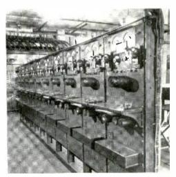
Voice frequency carrier telegraph terminal equipment at Pittsburgh
