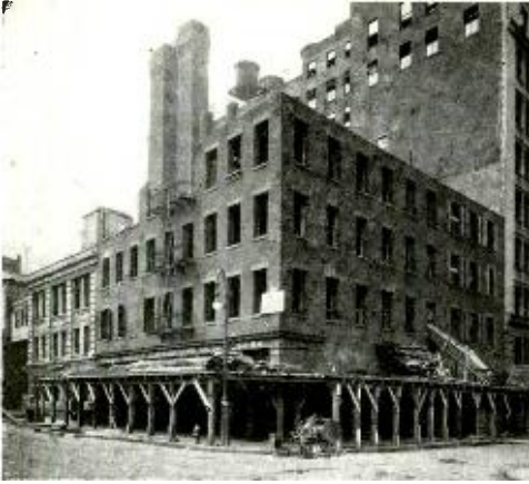
The old liquor warehouse partly demolished
