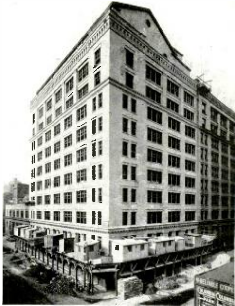
In August the outside brick work was completed
