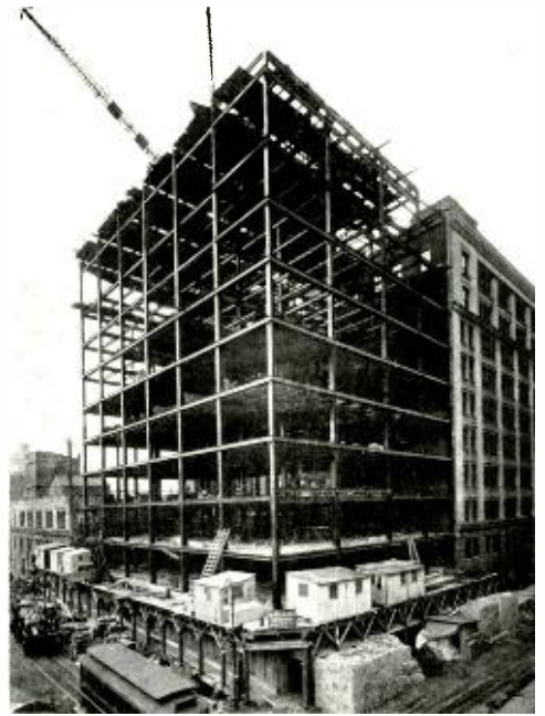
The steel framework as it appeared last April
