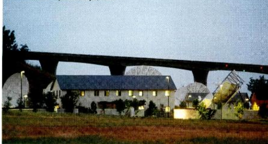
Teleport Access Systems is tapping a two-way satellite-based link through PanAmSat's teleport in Napa, Calif.
