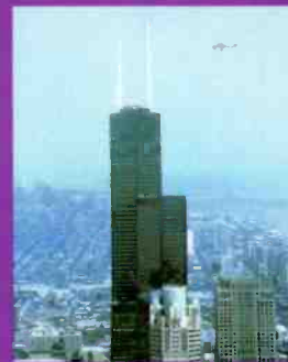
Fox's WFLD is the first to install its DTV antenna atop the Sears Tower.
