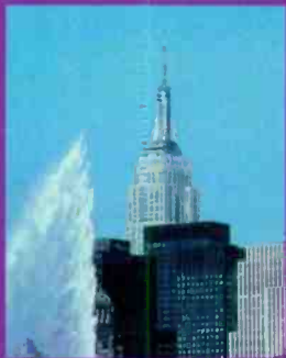
WCBS-TV and Fox owned WNYW have digital antennas atop the Empire State Building.
