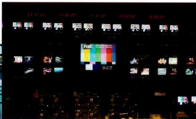
The project unites Fox Broadcasting Co. and 20th Century Fox in a single facility. The master control room is shown above.
