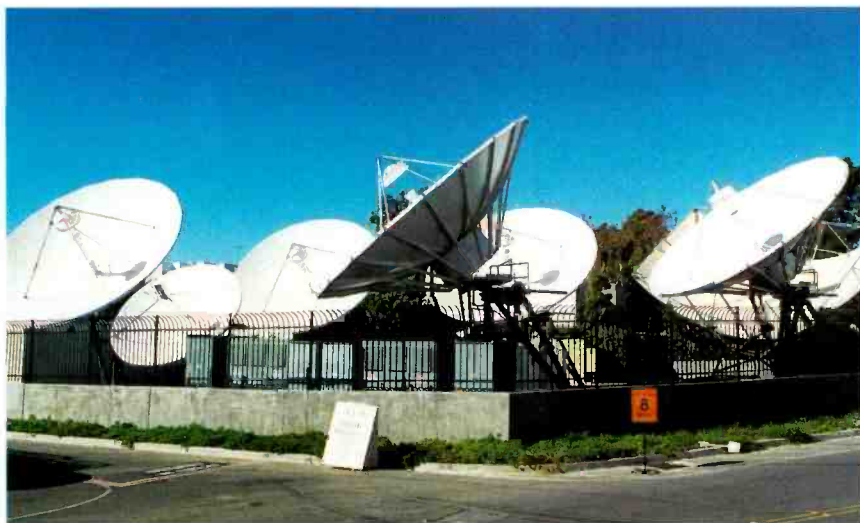
Adjacent to the new digital Fox Network Center is a multi-dish satellite uplink, which has been beaming Fox's prime time schedule to affiliates for more than a year.
