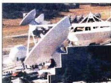
The Castle Rock Broadcast Center will uplink programming to the DBS-1 satellite. / 52
