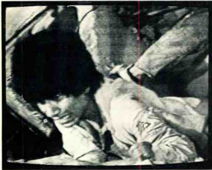
Pulling survivors from the debris
