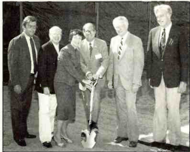
Going up. Blair Broadcasting of California's KSBW-TV Salinas, Calif., has begun construction of a new $4-million studio, office and production facility. The building will cover 34,000 square feet and will be built in two phases. The first, consisting of studios, technical facilities and a newsroom, is scheduled for completion in December 1983, with business offices scheduled to be finished by the summer of 1984. Shown at the ground-breaking ceremonies are (l-r): John F. Ryan, VP, and manager, Blair Television, San Francisco; John Fiedler, co-star, NBC-TV's Buffalo Bill; Barbara Shipnuck, Monterey county supervisor; Keith H. Moon, president, Blair Broadcasting of California and general manager, KSBW-TV; Salinas Mayor James E. Barnes, and John Thackaberry, VP and manager/NBC, Blair Television, Los Angeles.
