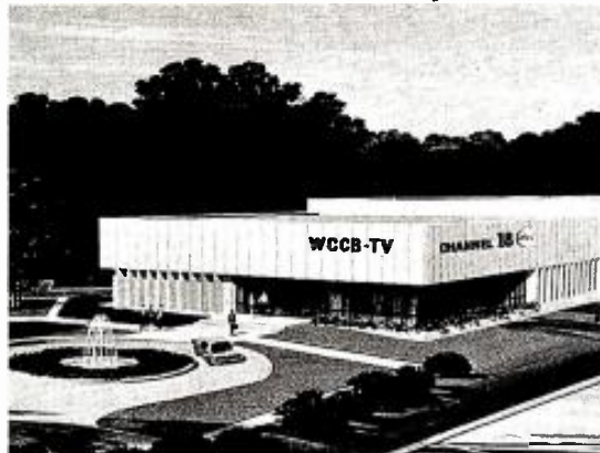
FLAGSHIP STATION AND CHARLOTTE HEADQUARTERS
