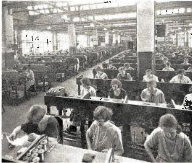
The Hawthorne Works of the Western Electric Company, scene of what one economist called "the most exciting and important study of factory workers ever made."
