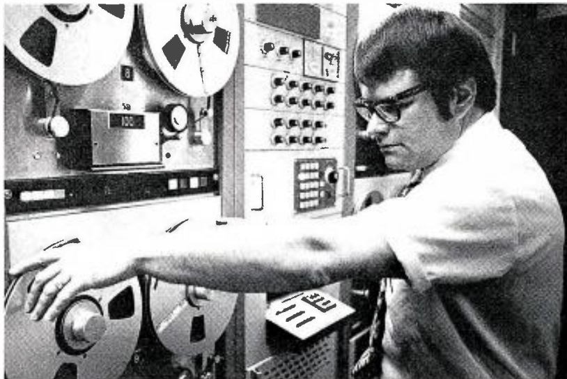
WBEN in Buffalo has designed and built probably the most modern broadcasting facility in America. And ITC is there with 9 open reel units and 37 cartridge machines!
