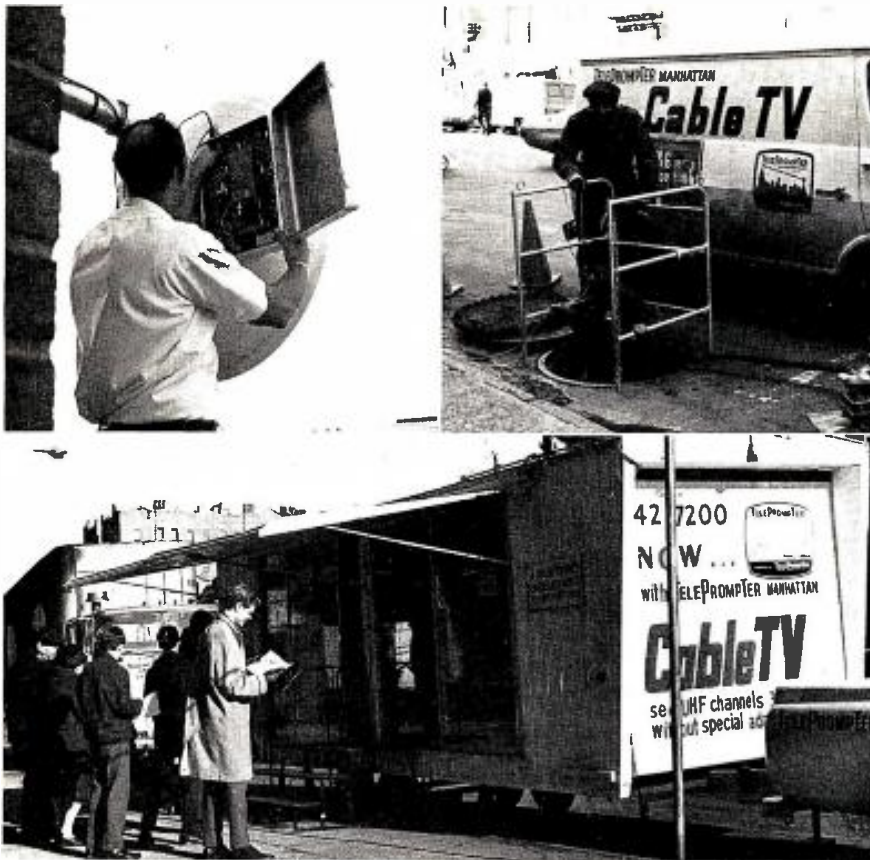
Three views of cable in Manhattan: On the roof of its 178th Street headend (upper left), Teleprompter Manhattan is installing a Theta Com AML 12 GC microwave system, which will transmit cable-TV programming to two locations: 711 Amsterdam on the West Side, and 86th Street and York Avenue on the East Side. The installation will shorten the amplifier-cascade length of Teleprompter's cable. Upper right: cable-TV technicians laying cable in the Upper Manhattan ducts of the Empire City Subway Co. Bottom: Mobile vans, hooked into Teleprompter's system, try to sell New Yorkers on the advantages of cable.
