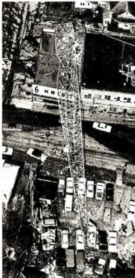
One of the first reports from the areas of the South devastated by Hurricane Celia last week was that the 145 mile-per-hour storm had flattened the tower of KRIS-TV Corpus Christi, Tex., knocking the station off the air. The structure was wrenched from its position on the roof of the station (top in photo) and strewn over the auto lot across the street. Communications with the storm-struck area were only partially restored by last Friday (Aug. 7) and no estimate of damages was available.
