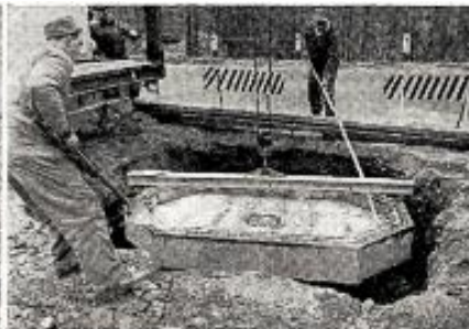
Lower manhole vault ...
