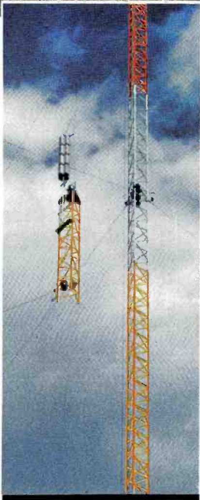
4 Antenna, mounted atop the top tower section, begins journey — up.
