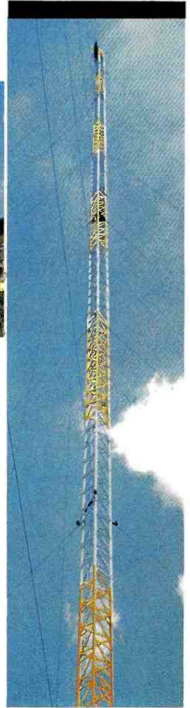
3 ROHN tower is shown erected and ready for antenna installation.
