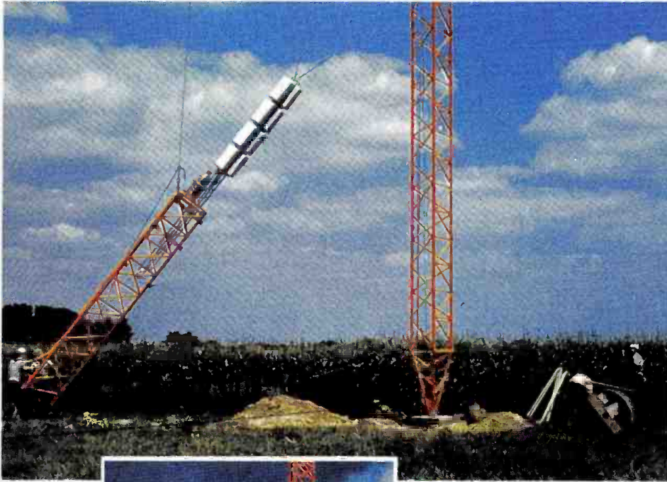
4 Antenna, mounted atop the top tower section, begins journey — up.
