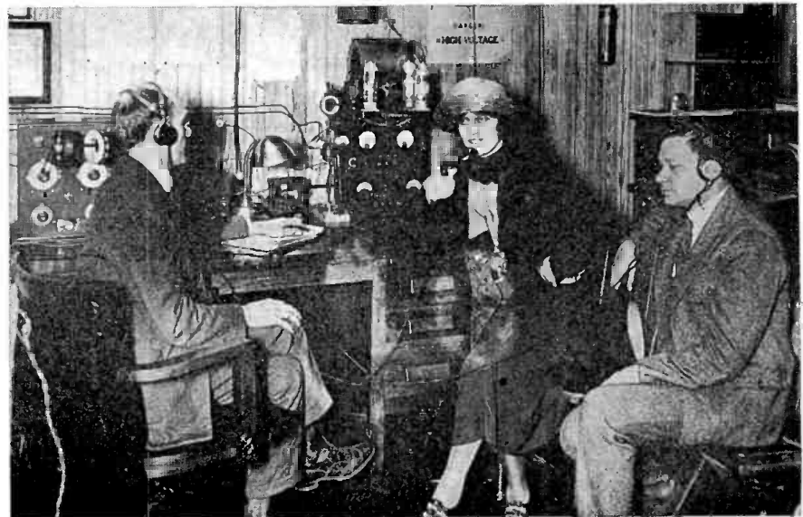
The facilities of WSB Atlanta in 1922 impressed famed opera singer Alma Gluck and her husband Efrem Zimbalist, an accomplished musician. George Iler (l) was WSB's first chief engineer.
