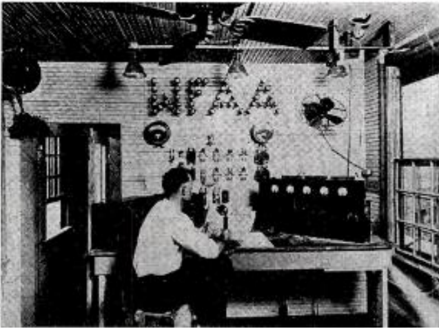
With this 50 watt transmitter, housed in a 9'x9' shed on top of the Dallas Morning News Building, WFAA Dallas went on the air in 1922.
