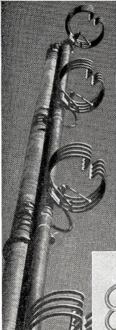
Above. Four sections of a BFA FM Antenna pole-mounted and interconnected by 3 1/8" coaxial transmission line.
