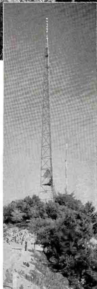
Designed for a 30-lb. wind load with 2" of radial ice, this 200' Ideco tower for KTTV atop Mt. Wilson supports a 6 bay channel 11 antenna.
