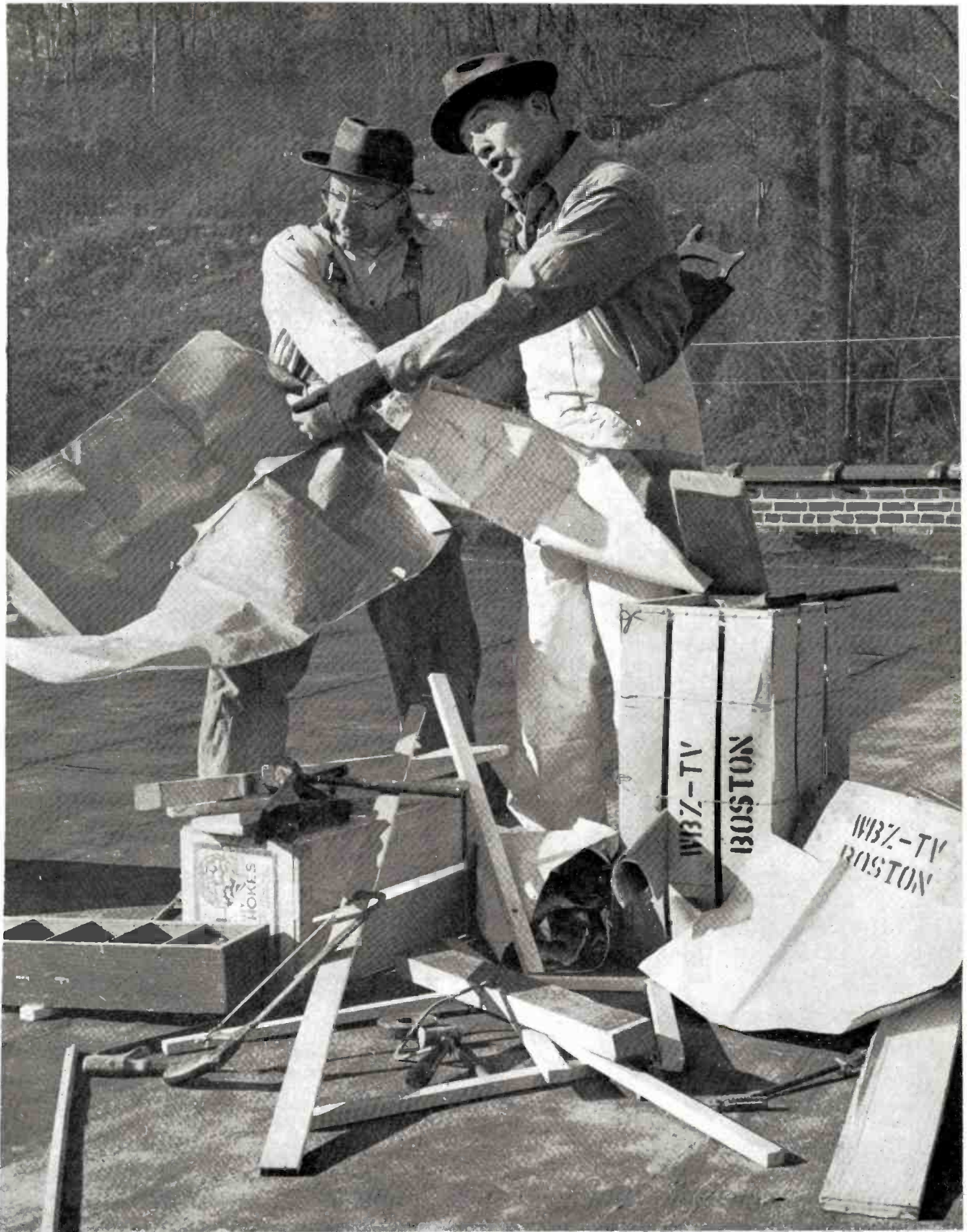
There's Something in the Air in Boston... Final Check of Specifications
