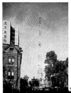
• That's just what WTOC-TV wanted . . . and Ideco tower engineers met this unusual requirement, neatly solved the problem of putting tower and transmitter building in the tiny area shown in the photo.
