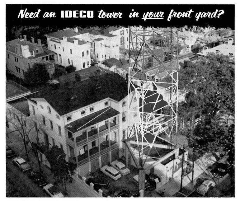
JOB DATA: Station WTOC-TV, Savannah, Ga. Self-supporting Ideco tower, 501 feet including 12 bay antenna, 40 lb. wind load. Transmitter building partially surrounds steel frame base for tower.
