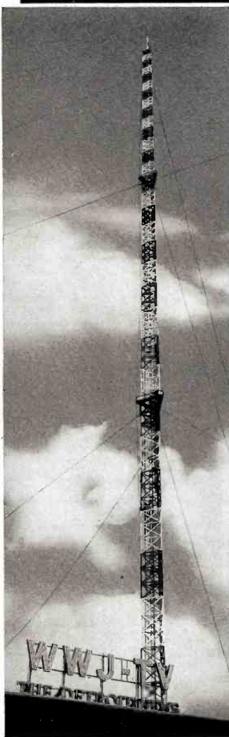
This 1063-ft. WWJ-TV tower serves the Detroit area. Weighing 265 tons, this typical Blaw-Knox-Graybar installation supports a 102 ft. antenna and a built-in two-man elevator.
