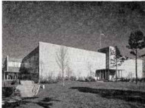
Pictured above is the $1 1/2 Million Jefferson Standard Broadcasting Company building. Operating from these kingsize facilities, WBTV serves more than 500,000 television families in its 100 UV/M area!
