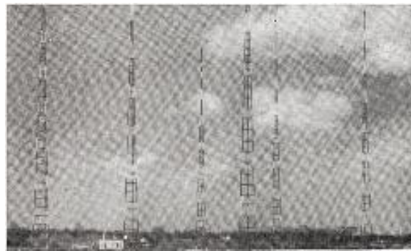
WFMJ-FM—Truscon Self-Supporting Directional Towers 400-Feet Tall
