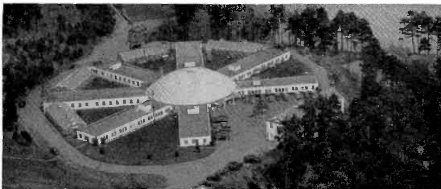
There's a Steel Hotel in Georgia. It's built like a wheel, with a 1500-seat auditorium for the hub. The wings radiate like spokes of the wheel, so that every guest has an outside room. Steel construction allows greater comfort per dollar of cost.
