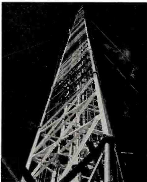
CLOSEUP showing construction details of WWJ-TV Detroit tower from Blaw-Knox.
