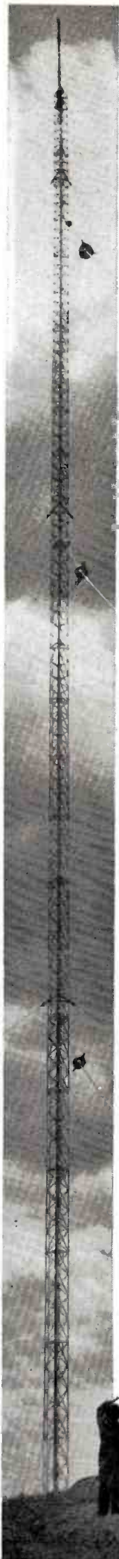
Massive 800-foot insulated tower for TV and FM radio
