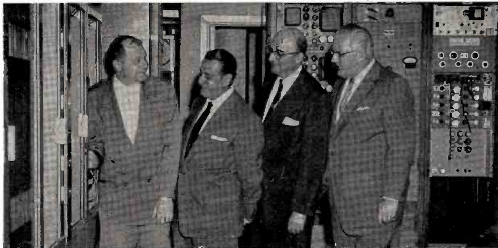
WAAM (TV) Baltimore executives inspect the station's new half-million-dollar wing and top-power tv transmitter. L to r: Ben Wolfe, engineering director; Norman C. Kal, WAAM Inc. executive vice president; Ben Cohen, WAAM Inc. president, and Ken Carter, WAAM general manager.
