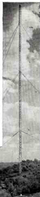
Slender 275-foot insulated tower for AM radio
