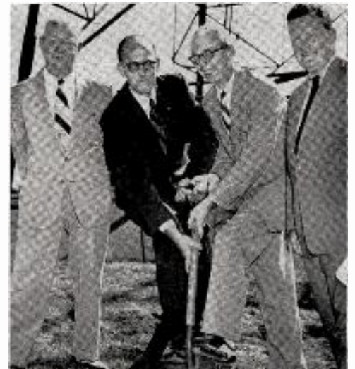
SHARE-TIMERS share spade in breaking ground for transmitter building. Executives of WHEC and WVET Rochester, both granted vhf Ch. 10 there on a share-time basis, expect to complete building in 60 days. At the task are (l to r) Clarence Wheeler, WHEC vice president; Irvin F. Lyke, WVET president-general manager; C. Glover DeLaney, WHEC general manager, and Paul C. Louthier, WVET vice president. In background is WHAM-TV TV tower, which also will be used by WHEC and WVET.
