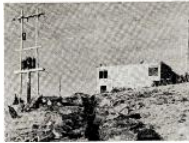
KXLY-TV transmitter building now under construction. ➤
