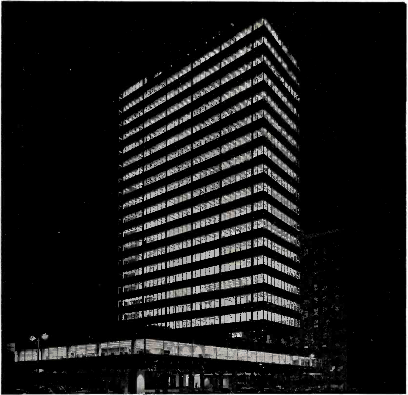
The 3542-ton steel frame for Lever House was fabricated and erected by Bethlehem. Architects: Skidmore, Owings & Merrill; Structural Engineers: Weiskopf & Pickworth; General Contractor: George A. Fuller Company.
