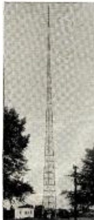
WTCH, Showano, Wisconsin. Truscon Self-Supporting Tower, 240 feet high.
