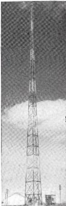
KAA-284, Owatonna, Minnesota, Northern Natural Gas Company. Truscon Self-Supporting Tower, 260 feet high.
