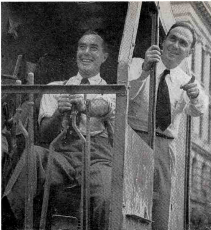
"AT WORK," Bob Swezey (l), general manager, and Edgar Stern Jr., president, of WDSU (AM-FM-TV) New Orleans, move full steam ahead at scene of construction of station's half-million dollar studio plant which will house all three facilities. It is scheduled for completion by early spring next year and will be directly adjacent to the administrative building.
