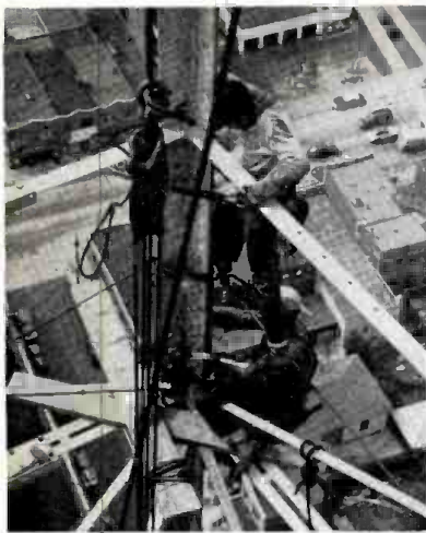
TOP MEN in their profession are Eddie Melley (upper figure) and Buddy Speir as they tighten bolts at 450-ft. level of WOR-TV New York's tower under construction at North Bergen, N. J. When completed, tower will be 760 ft. high.
