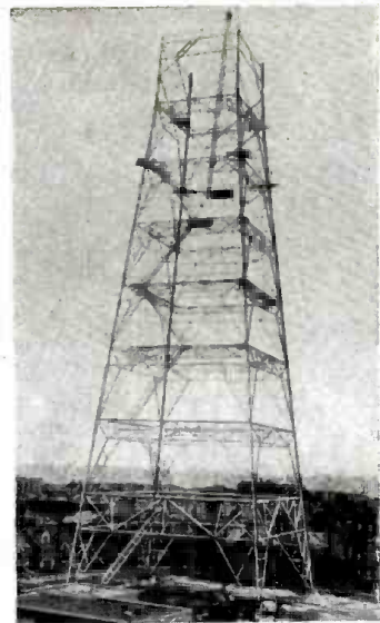
WOR-TV's Tower Construction
