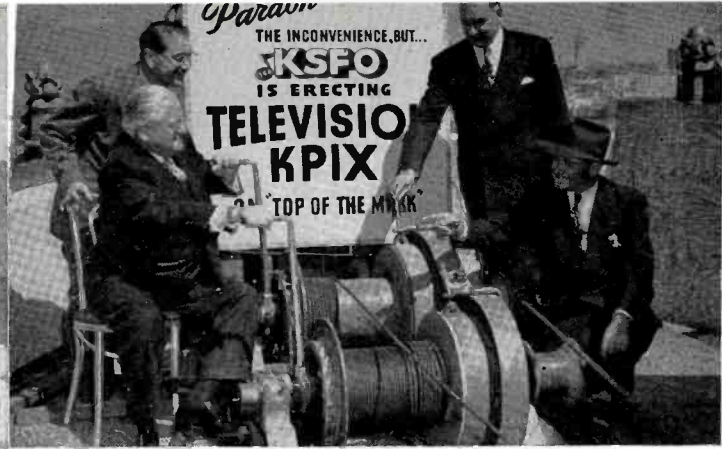
A NEW ANGLE on "ground-breaking" ceremonies is offered by KPIX, TV station for KSFO San Francisco. Mayor Elmer Robinson (seated) operates the winch that hoisted the 100-foot antenna to "Top of the Mark." Honorary steel riggers are (l to r) Philip G. Lasky, KSFO v.p.; Wesley I. Dumm, president; Paul Shepard, construction engineer.
