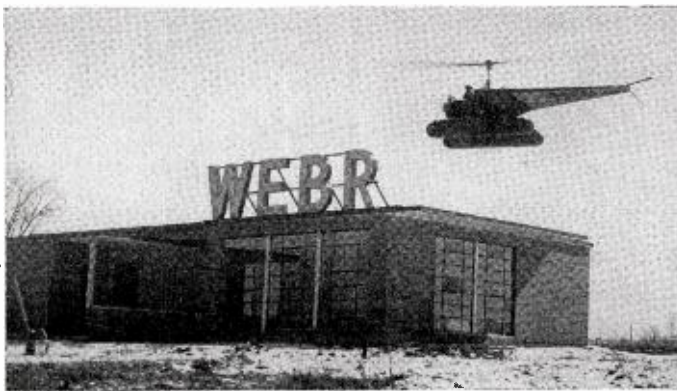
A NEW WAY to make field intensity measurements gets a tryout from WEBR Buffalo, using this helicopter. Edward S. Robinson, who flew the plane, is president of Helicopter Aircraft Service, Syracuse, and former assistant to WSYR president. A WEBR consulting engineer flew with him on the trip, and both agreed it will soon be possible to run complete field measurements in one day.
