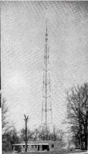
GRACEFUL tower and antenna of WSIX-FM Nashville rises to 292 feet, and is on a hill 1,110 feet above sea level. Station, owned by WSIX Broadcasting Co., increased its radiated power to 7½ kw April 9.
