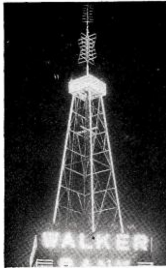
KDYL's super turnstile or "bat wing" antenna. Tower is outlined with red neon tubing.
