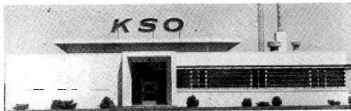
New KSO Building
