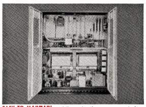
EASY TO MAINTAIN ::: full-opening doors, open vertical arrangement of components and power outlets, facilitate inspection and maintenance. All access doors are electrically and mechanically interlocked for safety of service personnel.
