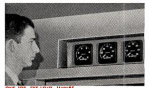
**ONE-JOB**, EYE-LEVEL METERS ... new 270° circular scale meters are at eye level for easy reading. Each instrument operates in but one circuit, eliminating instrument switching.
