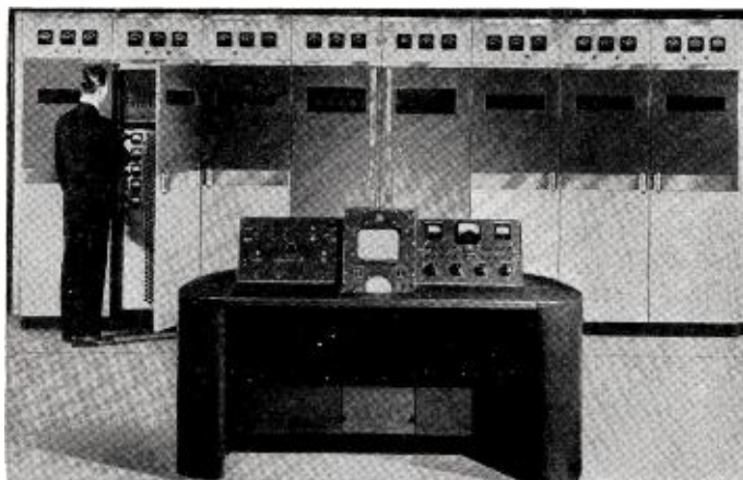
RCA's first postwar 5-kw television transmitter, Type TT-5A
