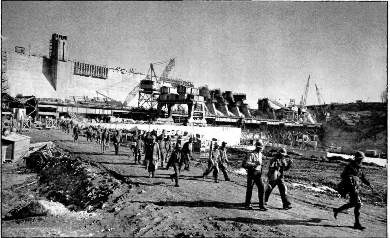
RECORD-BREAKING workmen change shifts at TVA's ██████ Dam, the vital wartime hydro-electric project which began storage of water on February 19, 1943.
