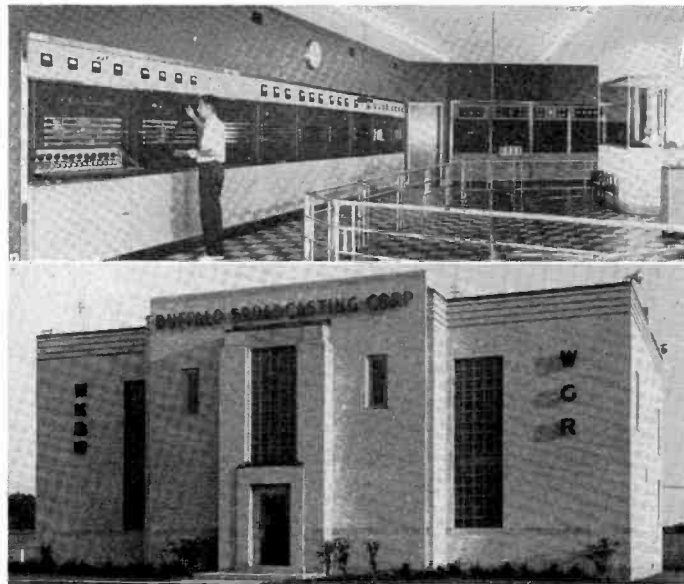
NEW $350,000 PLANT of Buffalo Broadcasting Corp., accommodating both WGR and WKBW, was formerly dedicated Oct. 30. Power of WKBW now is 50,000 watts and the station has carried CBS programs since Sept. 28. WGR is an MBS outlet. The WKBW transmitter panels (top left) extend 36 feet, with the WGR transmitter in background (right).
