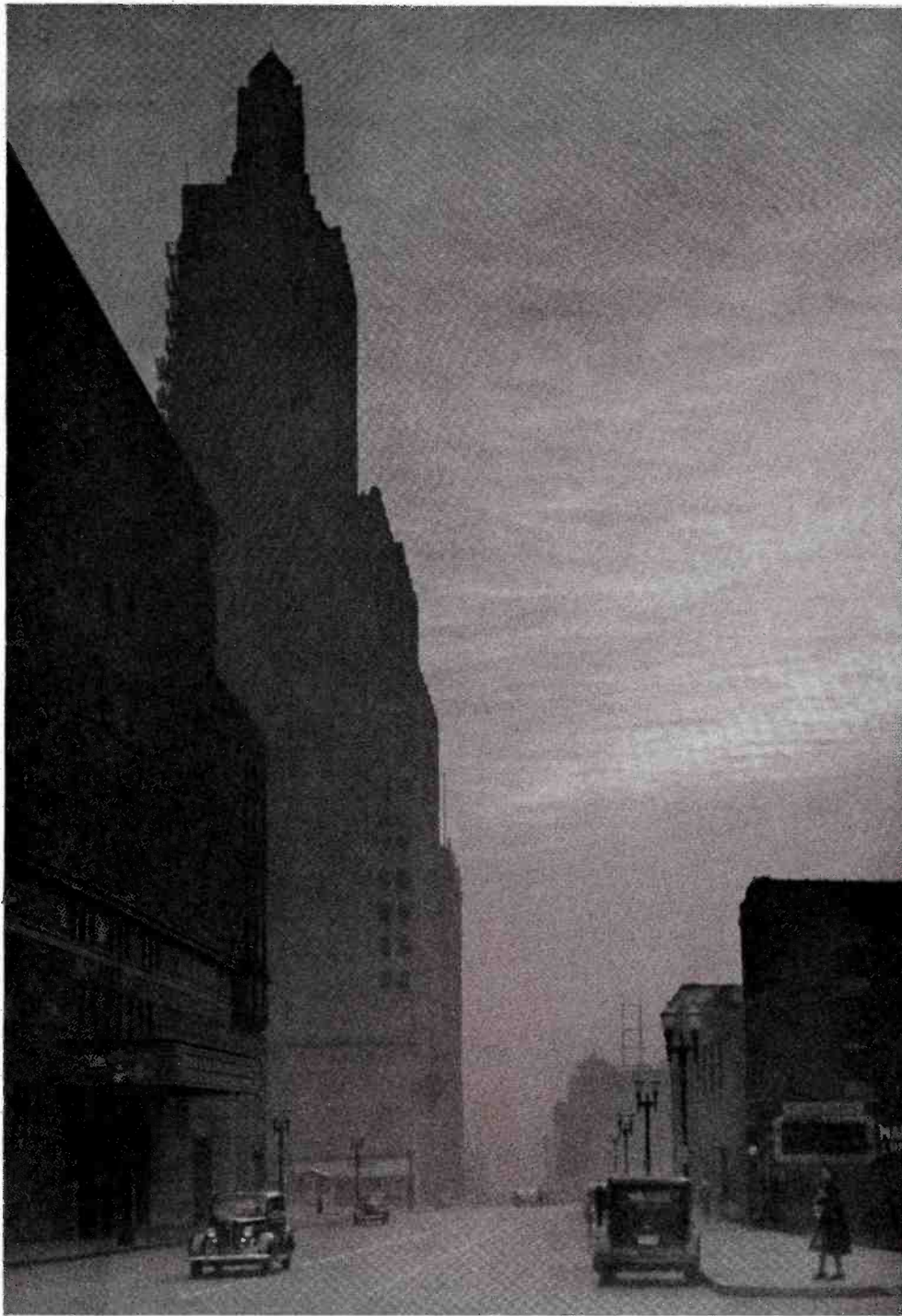
This photograph by D. D. Clarke was "shot at sunrise" on Fourteenth Street in Kansas City, Missouri. At left, foreground, is the Exhibition Hall of the city's new $6,000,000 Municipal Auditorium. In the distance, at left, is the magnificent skyscraper of the Kansas City Power and Light Company, Missouri's tallest building.
