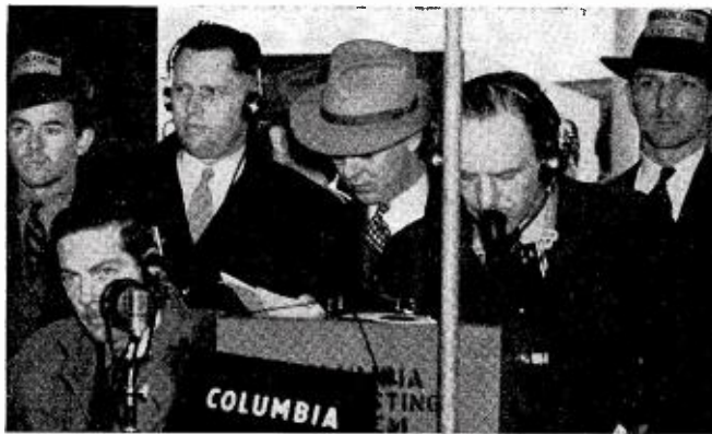
WHEN the Golden Gate International Exposition officially opened last month, the networks were there to cover the event for a nationwide audience. Here a CBS crew is standing by for the pickup from the bomber circling over Treasure Island. Seated is Paul Pierce, CBS producer. Standing (l to r) are Bob Garred, announcer; Fox Case, CBS Pacific director of special events; J. C. Morgan, KSFO program director; L. V. Howard, technical director, and Joe Walters, announcer.
