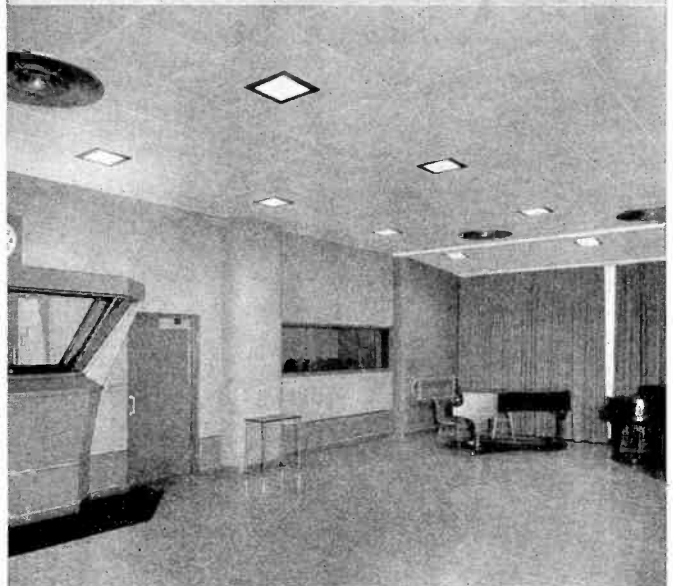
In the beautiful modern studios of Station WCCO, owned and operated by the Columbia Broadcasting System, effective sound control was obtained through the use of USG Perforated Surface acoustical treatment. USG Sound Insulation was used in floors, walls and ceilings, as well as between control rooms and studios.
