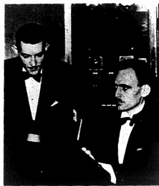
CBS Control Room in Detroit
