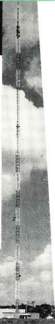
Typical EMSCO guyed TV tower Houston, Texas
