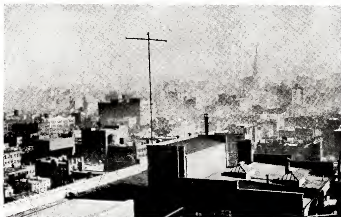
WEAF Antenna—1922. 463 West Street, New York City
