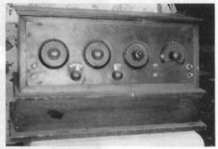
Figure 1. My Ozarka set as found. The tuning knob on the right is broken and the right-most selector switch is missing.
