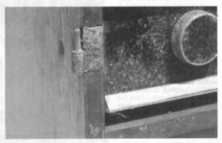
Figure 4. An example of damage to the wood, hinges, panel, and knobs can be seen here.
