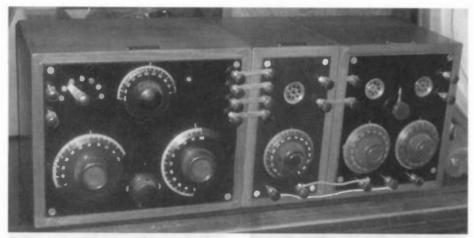
The three-panel "Cleveland Waves To You" set, shown above, sold for \$1,600. The panel functions are tuner, detector, and 2-step amplifier. An unusual item, this particular example was at one time in the Muchow collection. The nameplate, shown at right, is an artistic departure from the usual radio nameplate. The lettering superimposed over a wave-shaped line is: "wCALVEEVSETLOAYNODU."
